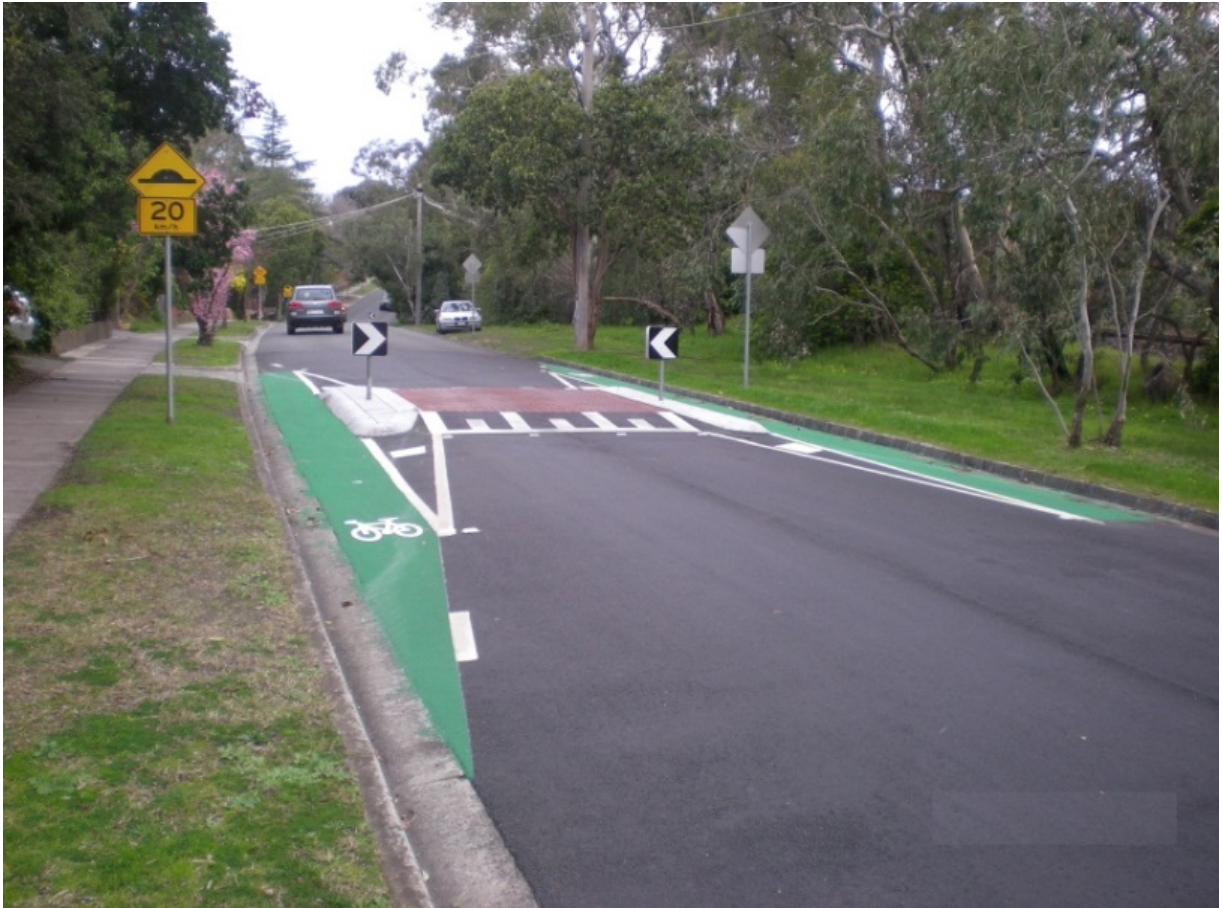
Figure 4.16: Example of good practice – cycle bypass of a road hump
