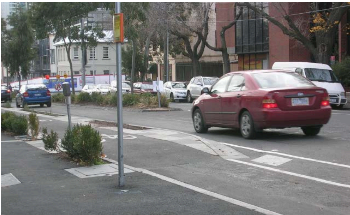
Figure 4.11: Kerb separated bicycle lane
