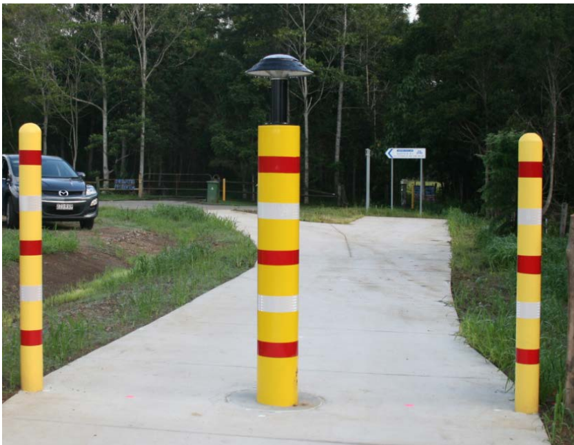
Figure 7.20: Example of a bollard treatment with lighting
