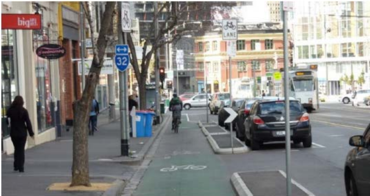
Figure 4.6: Separated bicycle lane with physical separation of parking
