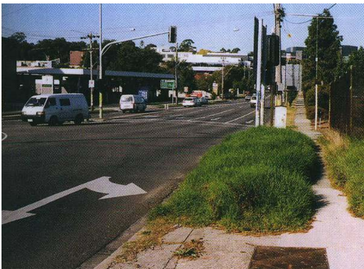
Figure H 1: The path to pedestrian signals is narrow and overgrown
