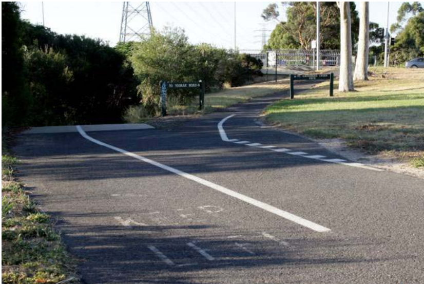
Figure H 2: The link path from Toorak Road joins at an acute angle, with restricted sight distance
