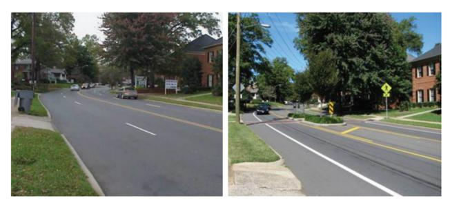
**Figure 5–3** Four-lane road in Charlotte, NC, changed to three-lane road with median turn lane to create space for bicycle lanes (Photos: Ken Tippette)
